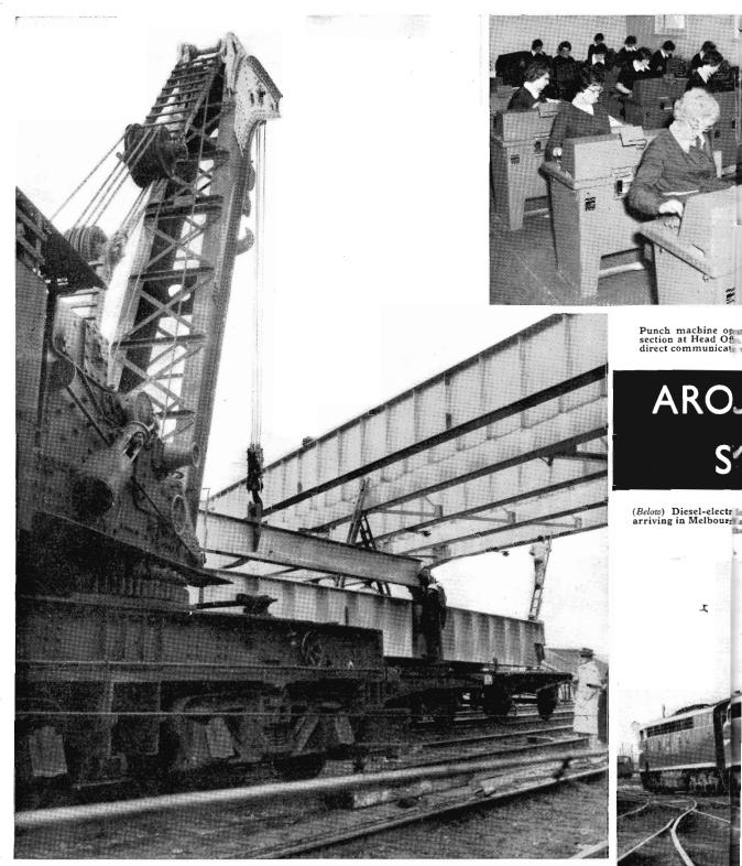
Eight ton girders for King Street traffic flyover being lifted into place by Victorian Railways 60 ton wrecking crane. The girders extend over the Port Melbourne and St. Kilda tracks.
