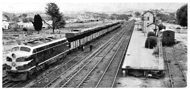
ABOUT to leave Bacchus Marsh station is one of the twice-daily brown coal laden trains, hauled by a B class diesel-electric locomotive.
