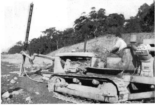
First ever used on the V.R. system, this air-driven rock drill—crawler-mounted with a forward boom for manouevring the\_drill into position—is helping between Wandong and Kilmore East to accelerate the standard gauge earthworks.
