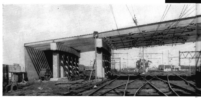
(Above) TAKING shape is this big grade separation job at Melbourne Road, Newport. Main span from 66 to 72 ft. long and 54 ft. wide, will take four lanes of road traffic. (Right) AFTEL
