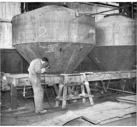
Apprentice Boilermaker working on construction of improved design 'X' type wagons for carriage of bulk cement. These wagons are so designed to permit loading both compartments simultaneously.
