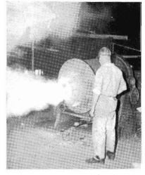
Operator checks rotary tilting furnace.
