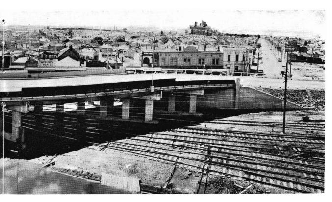
PICTURE shortly before being opened for traffic on October 3, this 1,400 ft. long overpass at Melbourne Road, Newport, eliminated a busy level crossing at the 'Down' end of the station. To help road traffic flow, roundabouts are being built at both approaches. Two subways will take pedestrian traffic.
