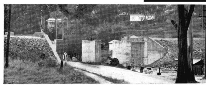
Belgrave line electrification : sub-structure for bridge over the main road at Upper Ferntree Gully.
