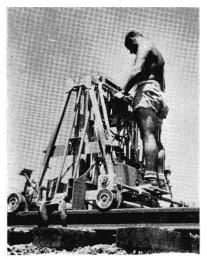
Track raised by Nordberg power track jack. Mechanization of track work on the Victorian Railways has trebled the annual mileage relaid while the cost per mile has been practically halved, compared with earlier hand methods.
