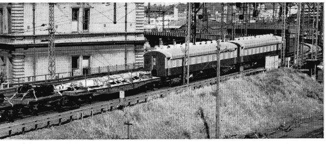
onwealth Engineering Pty. Ltd., at Dandenong as a Colombo Plan gift of the Federal Government to the Cambodian Railways, these two of 3 ft. 9 ins. gauge were pictured on their way for shipment from Appleton Dock. For the rail trip to the Dock, V.R. engineers superthe installation of temporary 5 ft. 3 ins. bogies to the vehicles; the 3 ft. 9 ins. bogies were carried on four flat K wagons.
