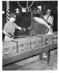
Pouring molten metal into moulds.
