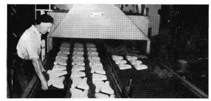
Loading cores for engine brake blocks on to the moving grate of the "Hurricane" core drying oven.
