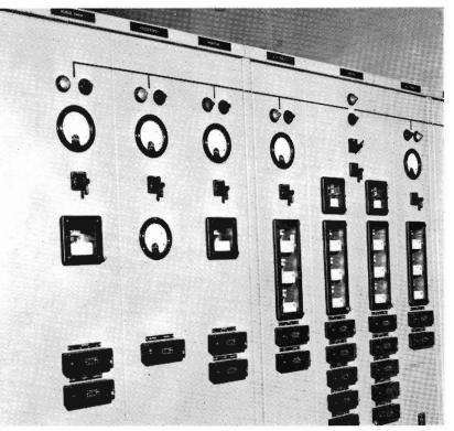
22,000 volt feeder control cubicles in a sub-station. Cost of a sub-station for a country line is about \$45,000; and the overhead from \$7,000 to \$10,000 a mile. These are some of the additional investment costs of electric locomotives that, except in conditions of very dense traffic, make them less economical than diesels.
