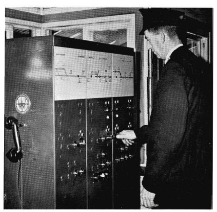
On the operating side, the greatest potential economies lie in further extensions of systems of automatic signalling and centralized traffic control. Assistant Stationmaster is operating C.T.C. equipment at Eastmalvern.
