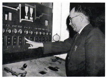
Control panel of sand conditioning installation which was designed and built at Newport Workshops.
