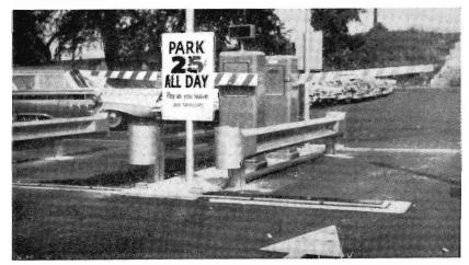
A commuter parking lot at Matheson, Illinois, has automatic gates installed. An approaching motor car trips a treadle to raise the entrance gates ; when leaving, the driver deposits a coin to open the exit. Installation is expected to pay for itself in  $2\frac{1}{2}$  years. [On the V.R. system, the motorist is not charged for leaving his vehicle in car parks—of which there are more than 70 at suburban stations. —Ed.]
