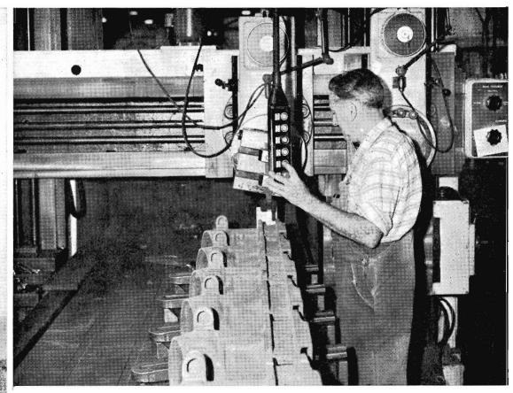
This Butler planing machine, with its 35-ft. table, is the largest in the Machine Shop at Newport Workshops. It planes the seats of 24 axle boxes in one operation. Iron Machinist Eric Jones is shown making final adjustments before starting the machine.
