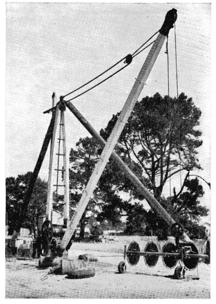
IMPORTANT in the overall efficient working of the Maffra goods yard is the six-ton capacity electric crane.
