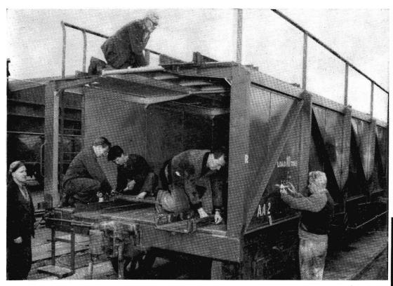
IMPROVED AA wagons for transporting motor cars have two special features: sides to obviate dust damage to cars and a roof totally enclosing the lower deck, so forming a floor for the upper deck that prevents oil dripping on to cars beneath. (Above) Fitting a wagon with motor car fastening gear. (Right)\_Twenty-four cars are loaded on these four AA\_wagons.
