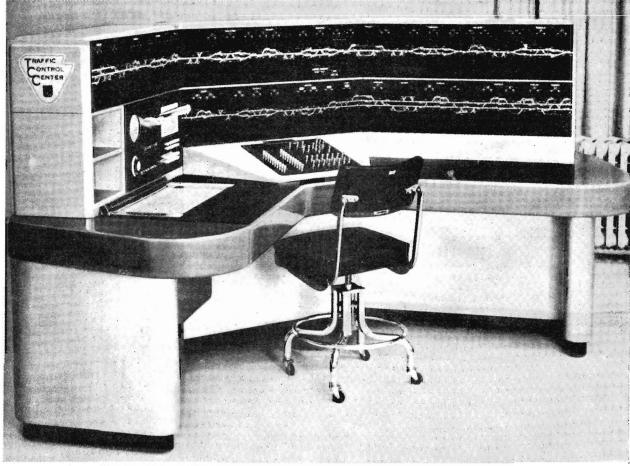
Traffic Control Centre showing 2-tier track diagram, communication switchboard, control panel and automatic train graph. The Centre for the standard gauge will be similar.
