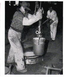
(Above) Removing crucible of aluminium from oil fired pit furnace before pouring into moulds. Aluminium is used to produce small fittings for carriages, etc.
