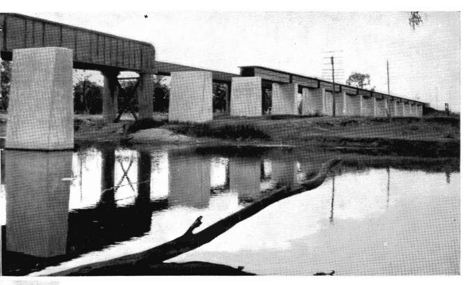
BRIDGE over Broken River, near Benalla. Concrete piers at the right will take standard gauge line. Steelwork on the approach spans supplied by N.S.W. Railways has been erected. The river spans are 63'; plate girders are now being fabricated for these.
