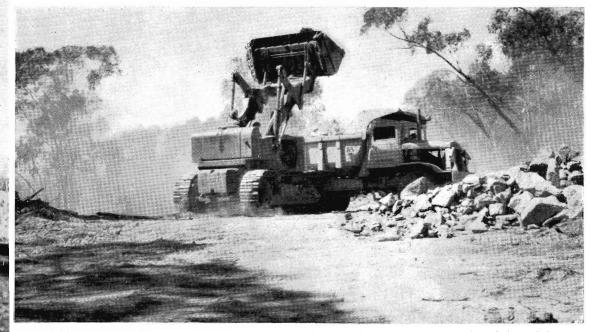
LOADING stone at Glenrowan for transport to crusher. To supply the 600,000 cubic yards of specially graded, crushed stone used for ballast, contractors have established crushing plants at Glenrowan and Barnawartha and more plants are being set up near Dysart and Euroa.
