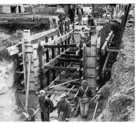
Form work being erected for the concrete retaining walls of the pedestrian subway that will pass under the tracks and road way at the Hampshire Road overpass, Sunshine. Estimated to cost £300,000, the overpass is one of the major grade separation projects in the metropolitan area.
