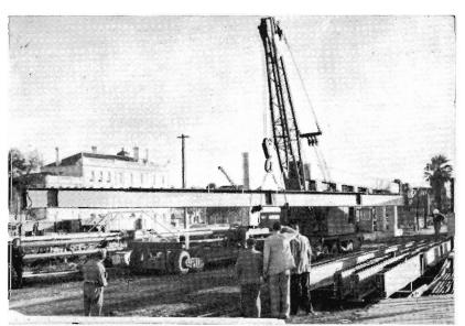
Lifting a girder for the new overpass at Melbourne Road level crossing, Newport.
