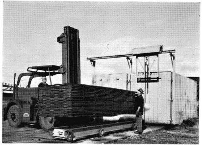
(Above) PLACING timber on the special hydraulic lift trolley that will move it into the treatment chamber where "re-conditioning" takes place. (*Right*) OPENING of the chamber door is effected by an over-head-conveyor lifting device that hoists the door clear of the slots, and then moves it laterally away from the chamber door-way. (*Below*) HAVING been treated in the steam chamber, the timber is about to be placed on the trolley for removal.
